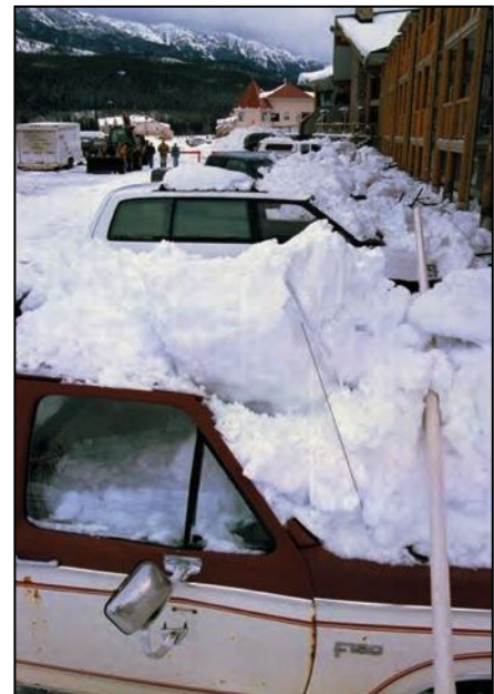
Figure 4: An example of the damage caused by snow build-up on roof forms
